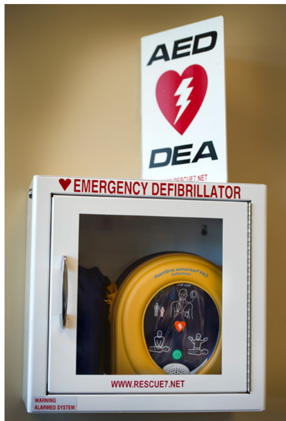
Automated external defibrillators are now in every building on Memorial's campuses
