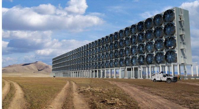
Figure 1: Banks of fans blow air through a carbon dioxide-capturing solution in this rendering of a direct air capture plant. Source: <https://www.science.org/content/article/cost-plunges-capturing-carbon-dioxide-air>
