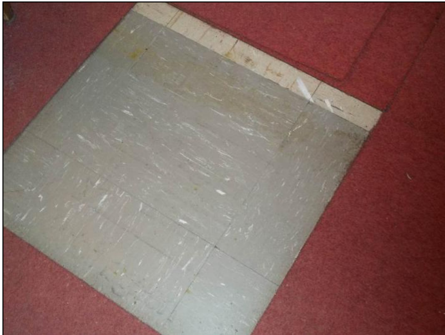
Photograph 7: Room SN1052. Asbestos containing 1' x 1' vinyl floor tile under carpet. Sample SN-66.
