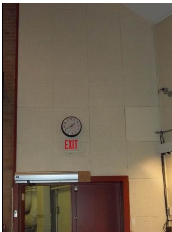
Photograph 18: Room SN2109. Asbestos containing transite panels. Sample SN-105
