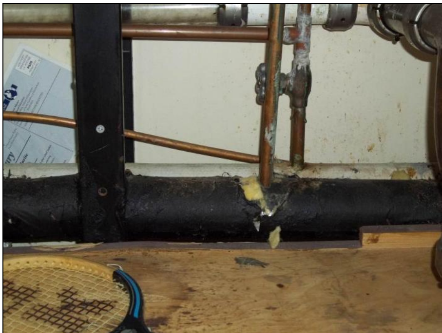
Photograph 22: Room SN4100. Asbestos containing tar mastic on fiberglass pipe insulation. Sample SN-133
