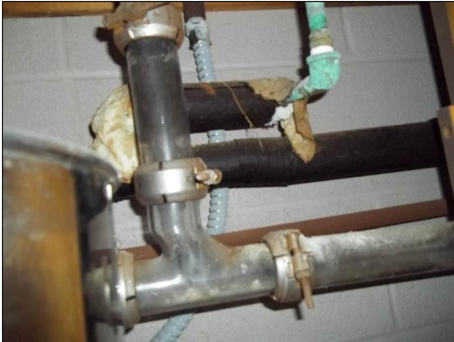
Photograph 36: Room SN4020. Asbestos containing pipe fitting insulation, located within a cupboard, in poor condition.
