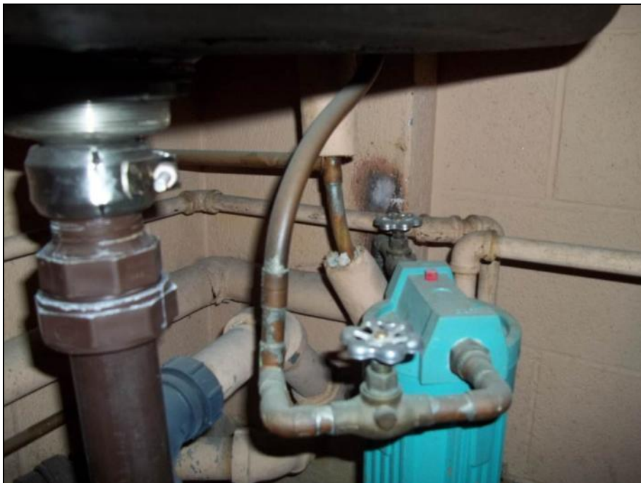
Photograph 31: Room SN3006C. Asbestos containing pipe fittings located within a cupboard, in poor condition.
