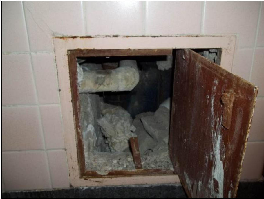
Photograph 6: Room SN1068. Asbestos containing pipe fitting insulation. Sample SN-61.
