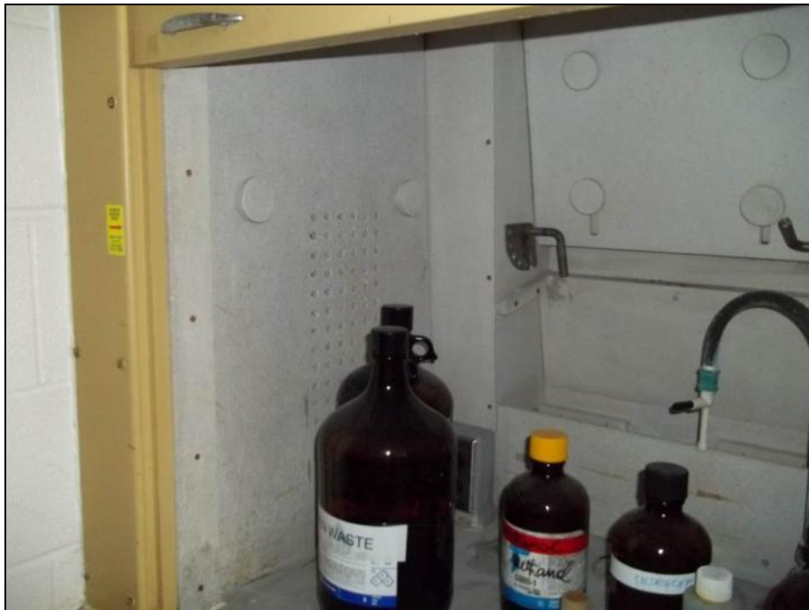
Photograph 27: Room SN1045C. Asbestos containing transite fume hood. Sample SN-12
