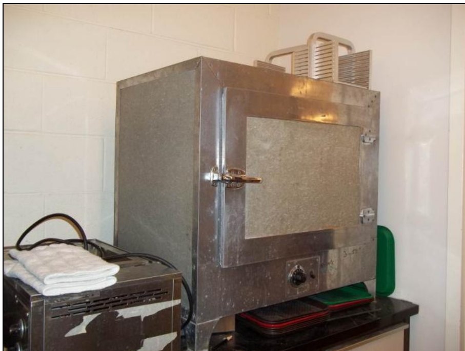
Photograph 43: Room SN4098. Suspect asbestos containing transite autoclave.
