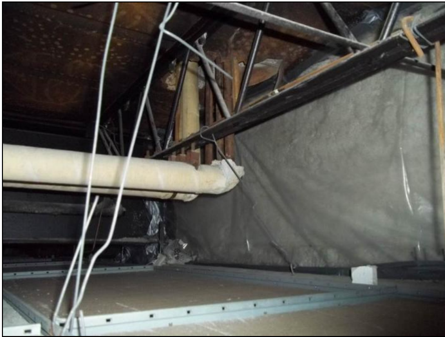
Photograph 30: Room SN3006B. Asbestos containing pipe fittings located above ceiling tile, in fair condition.
