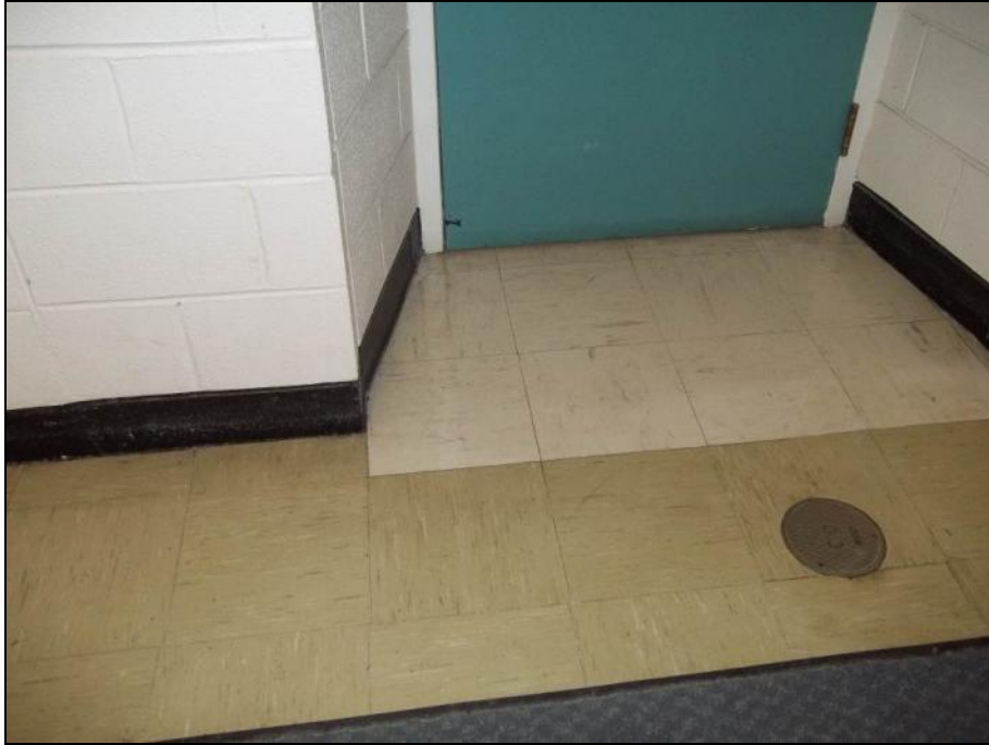
Photograph 24: Hallway SN1C03. Asbestos containing 1' x 1' green vinyl floor tile. Sample SN-03
