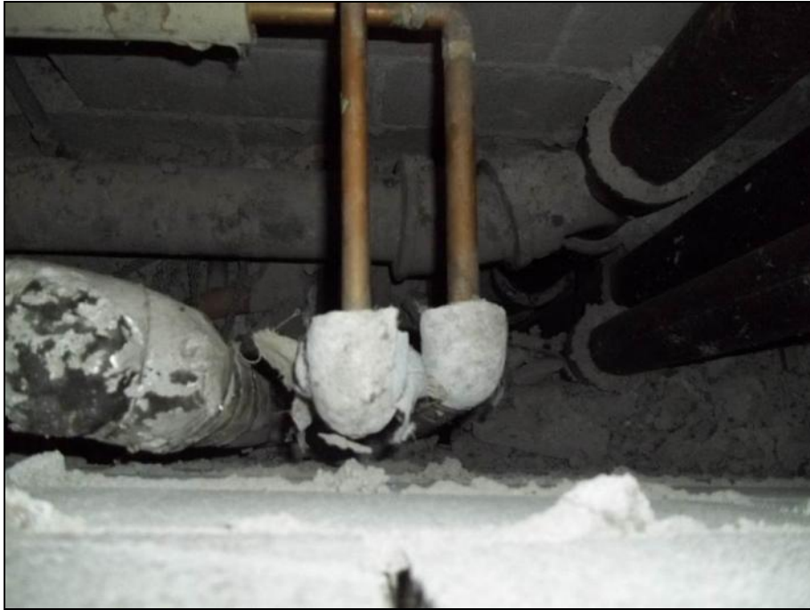
Photograph 34: Room SN4002. Asbestos containing pipe fitting insulation, located within a wall hatch, in poor condition
