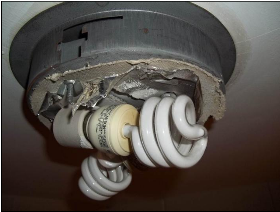
Photograph 28: Room SN1030. Asbestos containing light fixture heat shield. Sample SN-27
