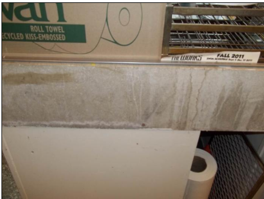
Photograph 15: Room SN3107. Asbestos containing transite on counter. Sample SN-89.
