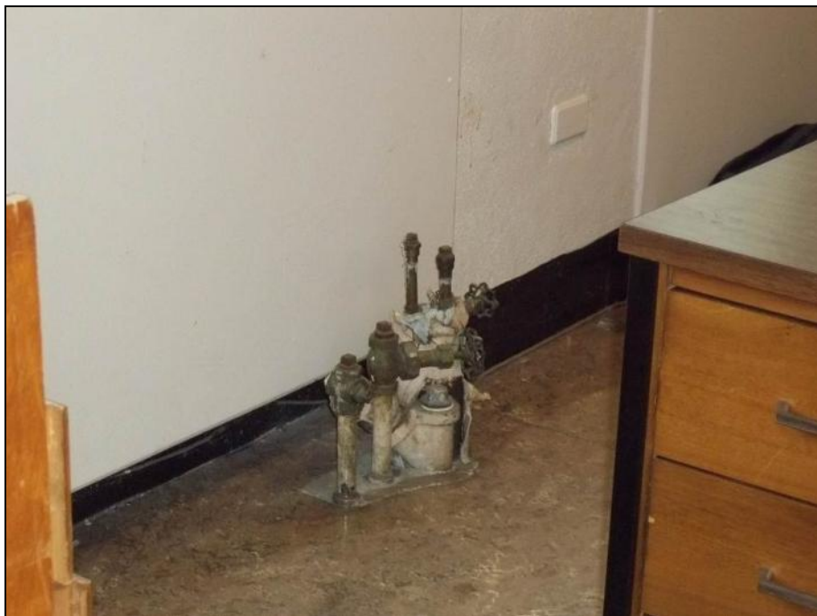
Photograph 41: Room SN3112A. Asbestos containing pipe fittings, in poor condition
