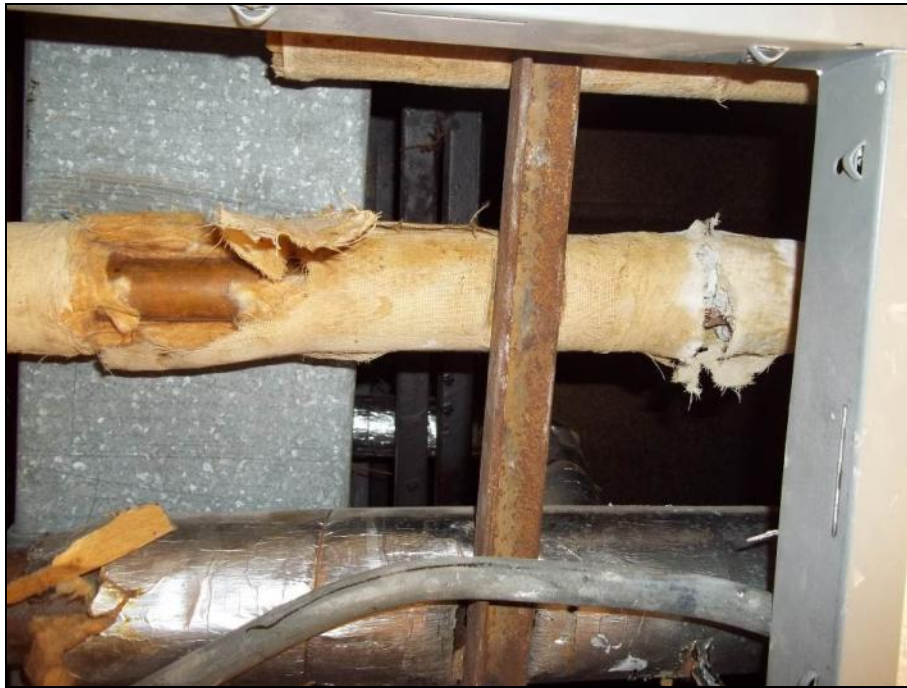
Photograph 42: Room SN1066. Asbestos containing pipe fittings, located in the ceiling space within an access hatch, in poor condition
