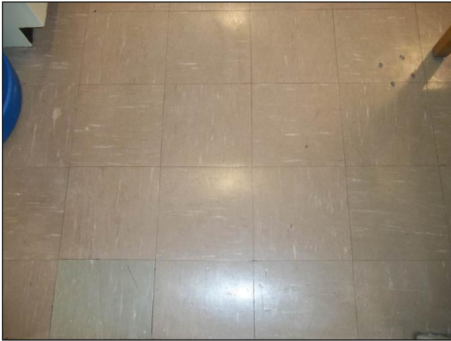
Photograph 3: Room SN1074C. Asbestos containing 9" x 9" vinyl floor tile and mastic. Sample SN-52
