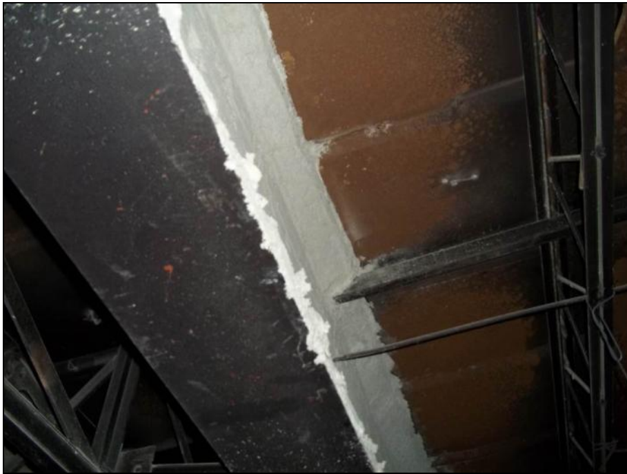
Photograph 16: Room SN3125D. Asbestos containing fireproofing on I-Beam. Sample SN-95
