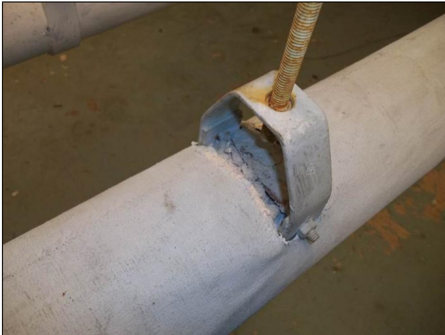
Photograph 21: Room SN2048A. Asbestos containing pipe hanger insulation. Sample SN-130
