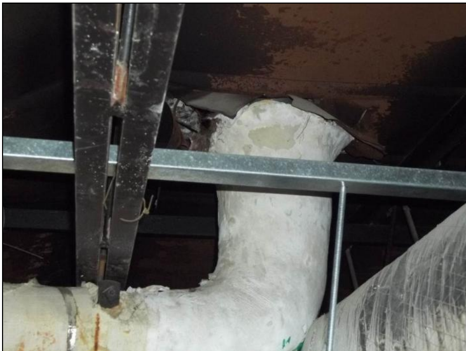
Photograph 33: Room SN4117. Asbestos containing rain water leader, in poor condition
