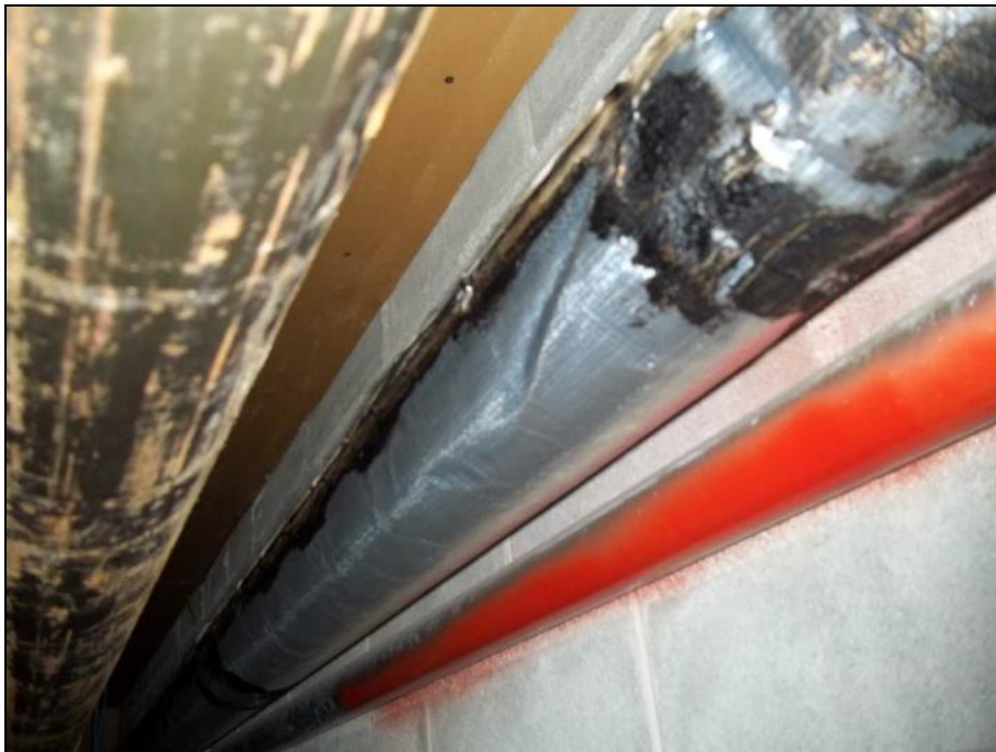
Photograph 29: Hallway SN2C03. Asbestos containing tar on fiberglass insulated pipe. Sample SN-29
