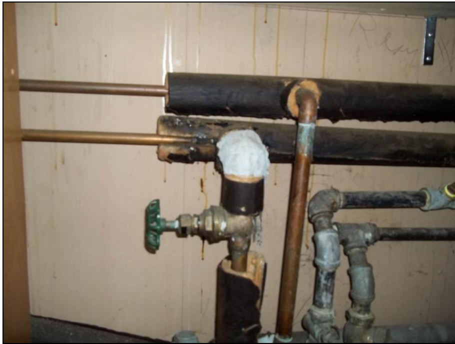
Photograph 40: Room SN3109. Asbestos containing pipe fittings, located within a cupboard in poor condition
