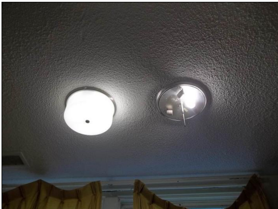
Photograph 13: Room SN2091. Asbestos containing light fixture heat shields Sample SN-79. Also note asbestos containing textured ceiling.
