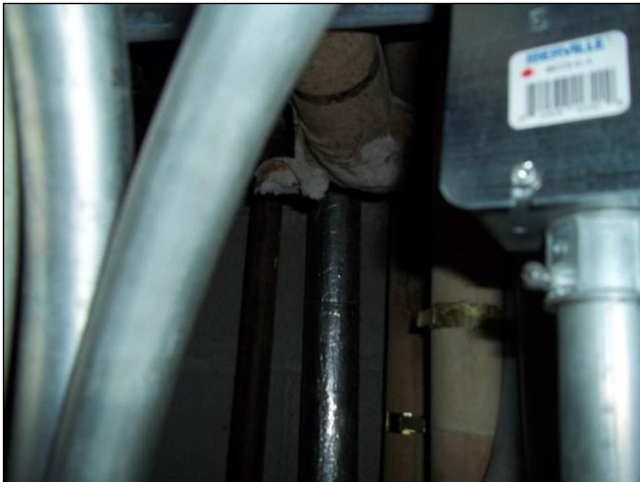
Photograph 47: Hallway SN3C02. Asbestos containing pipe fitting, in poor condition
