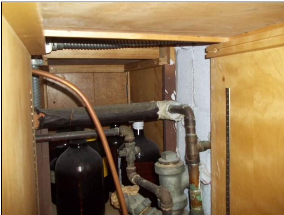
Photograph 35: Room SN4020. Asbestos containing pipe fitting insulation, located within a cupboard, in poor condition
