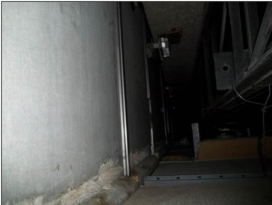
Photograph 37: Room SN3125D. Asbestos containing transite panels on the exterior wall, above ceiling tiles.
