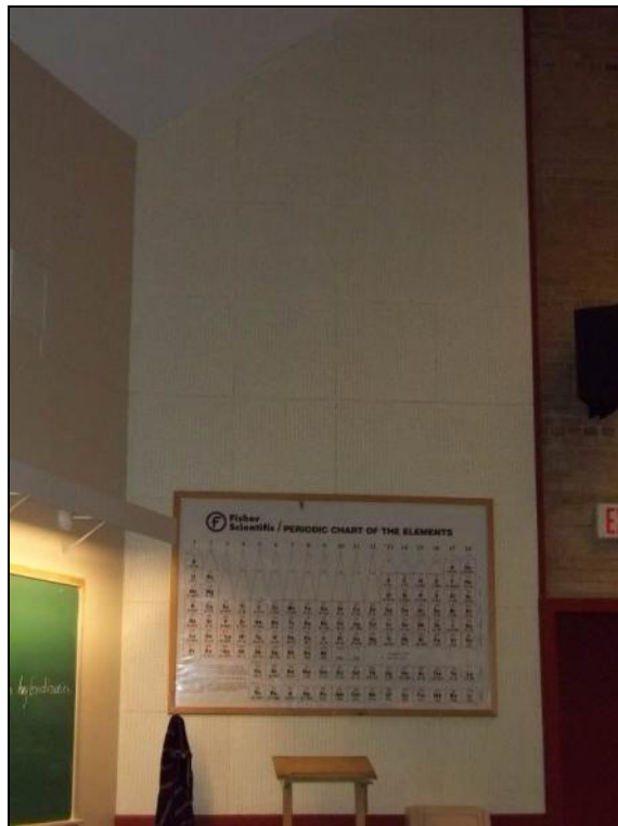
Photograph 17: Room SN2109. Asbestos containing transite panels. Sample SN-105
