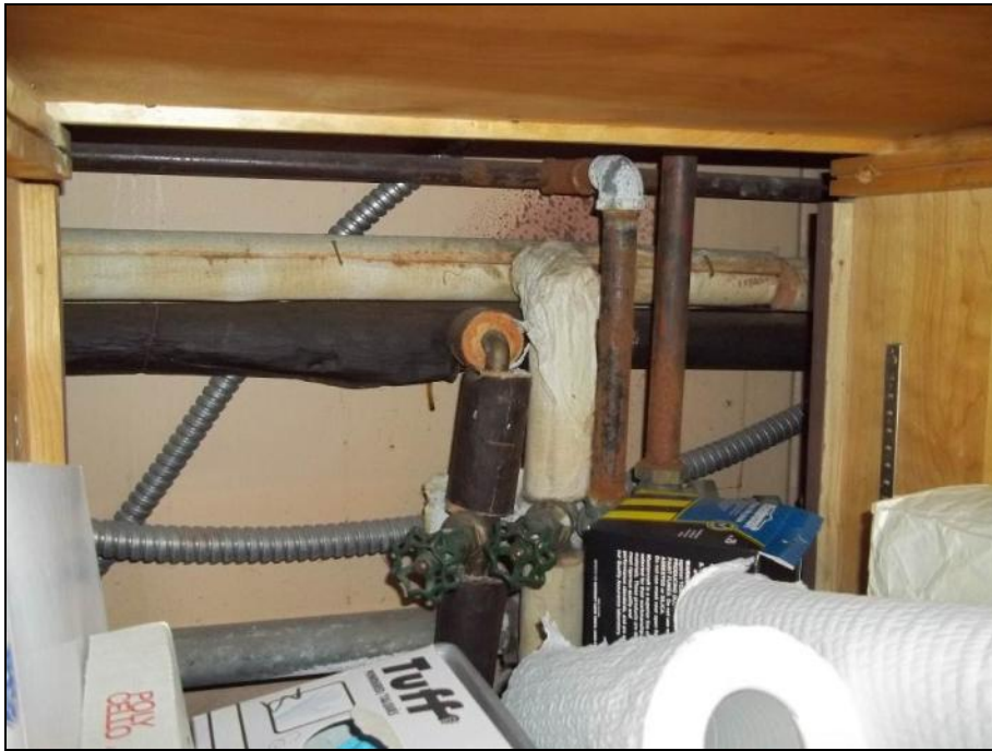
Photograph 38: Room SN2092. Asbestos containing pipe fitting, located within a cupboard, in poor condition.
