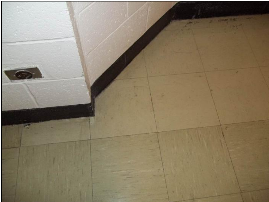
Photograph 25: Hallway SN 1C03. Asbestos containing 1' x 1' light green vinyl floor tile and mastic; and cream with brown. Samples SN-05 and SN-06.
