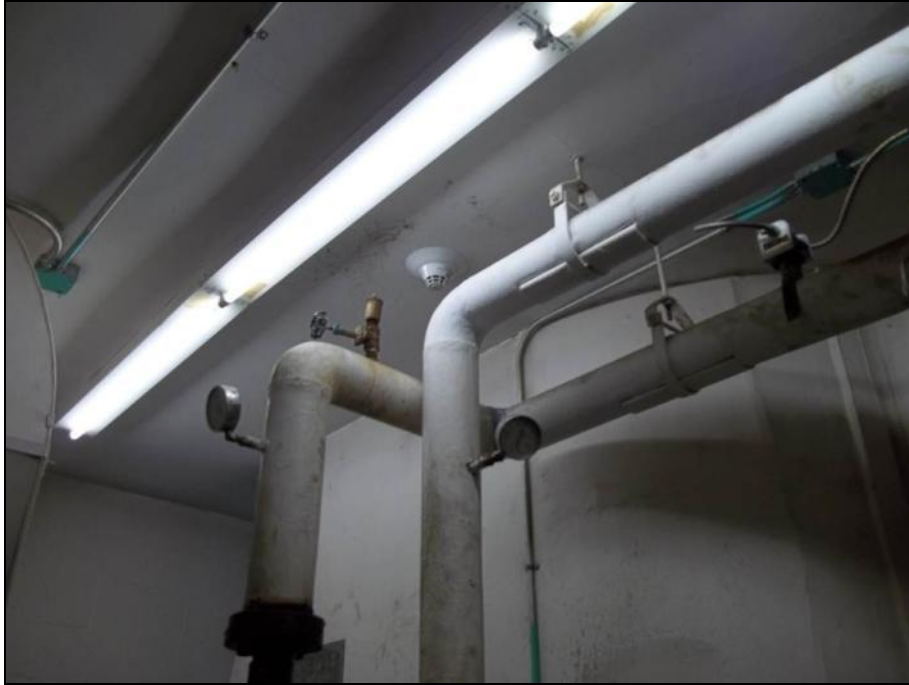
Photograph 20: Room SN4051. Asbestos containing pipe fitting insulation. Sample SN-128
