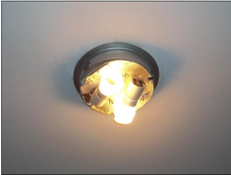
Photograph 44: Room SN4090. Asbestos containing light fixture heat shield, in poor condition
