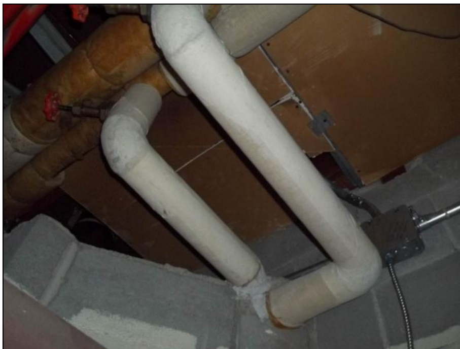
Photograph 23: Vestibule SN1V03. Asbestos containing pipe fitting insulation. Sample SN-02
