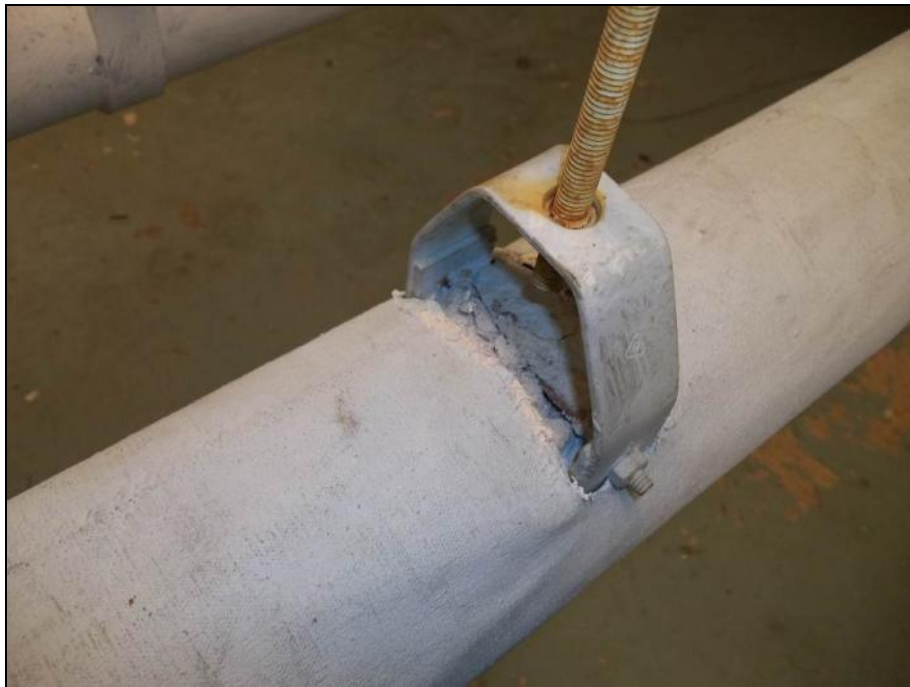
Photograph 45: Room SN2048A. Asbestos containing pipe hanger insulation, in poor condition
