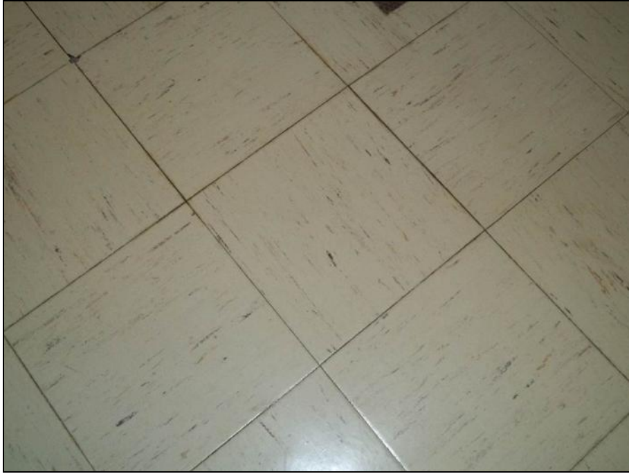
Photograph 1: Hallway SN1C04. Asbestos containing 1' x 1' vinyl floor tile and mastic. Sample SN-47
