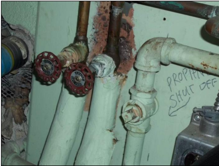
Photograph 32: Room SN3023. Asbestos containing pipe fittings located within a cupboard, in poor condition
