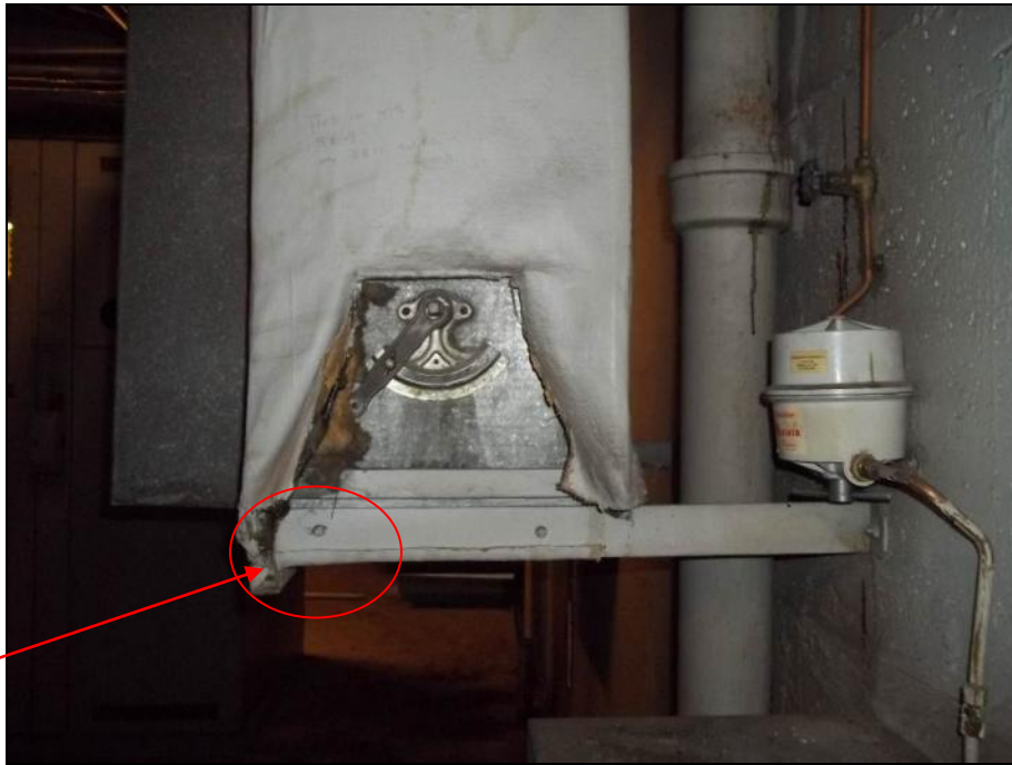
Photograph 12: Room SN1111. Asbestos containing parging along the seam of the fiberglass insulated duct. Sample SN-75.
