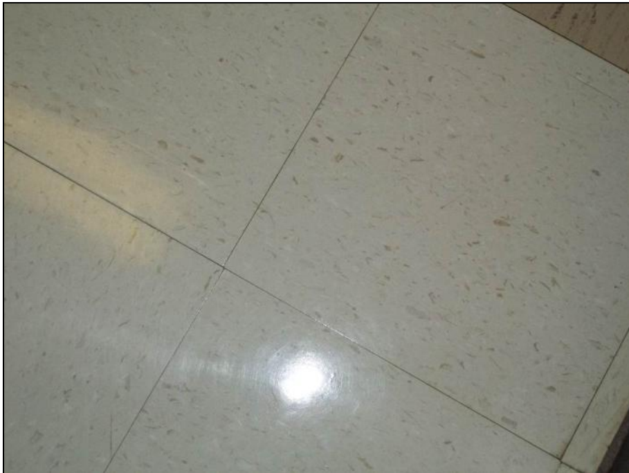
Photograph 2: Hallway SN1C04. Asbestos containing mastic under floor tile. Sample SN-48.
