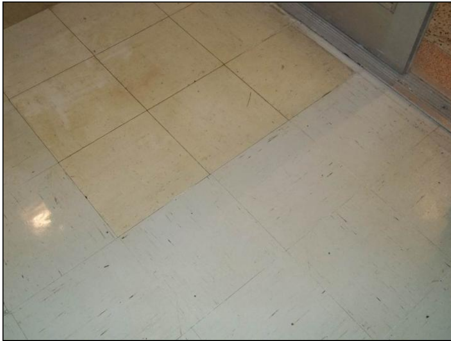
Photograph 26: Hallway SN1C03. Asbestos containing tile associated with grey tile. Sample SN-07.
