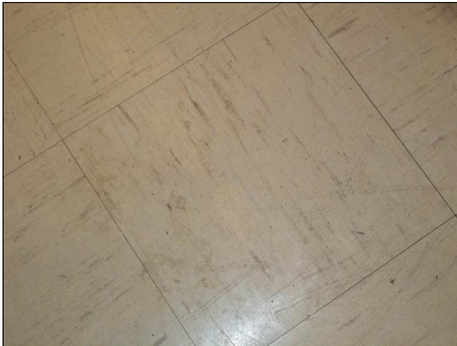
Photograph 8: Room SN1050. Asbestos containing 1' x 1' vinyl floor tile and mastic. Sample SN-67.
