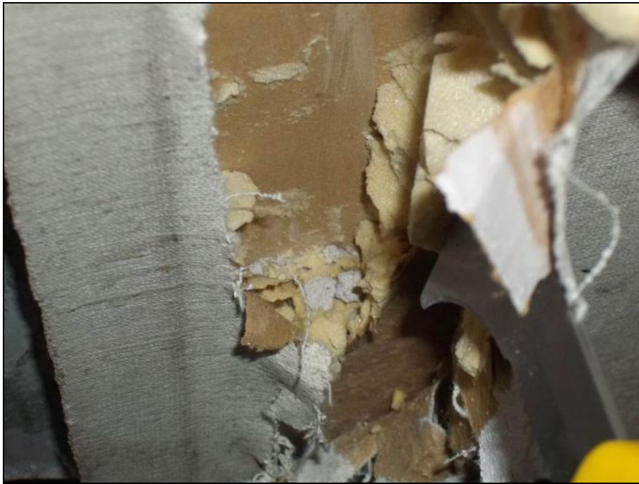
Photograph 14: Room SN2085. Asbestos containing padding debris on foam insulated duct. Sample SN-85.
