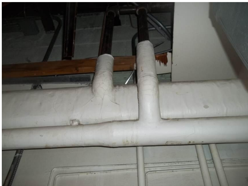
Photograph 3: Suspect linear pipe insulation in Room HD1011. The piping was too high to access for sample collection or visual inspection.
