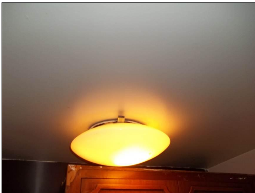
Photograph 7: Samples DH-19 and DH-20 as found in Room DH2006. The shield contained two layers, both were found to be asbestos containing.
