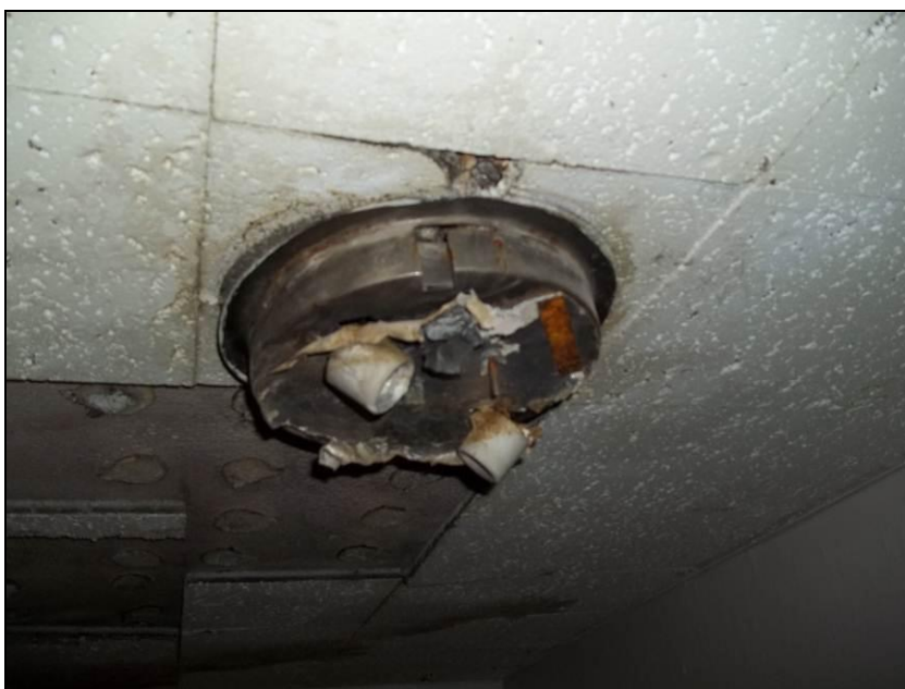
Photograph 8: Sample DH-21, of an exposed light fixture heat shield, in poor condition.
