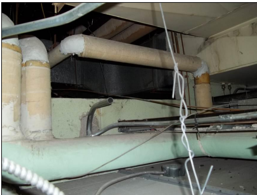
Photograph 1: Pipe fitting insulation in DH1010, above the ceiling tile, in poor condition.
