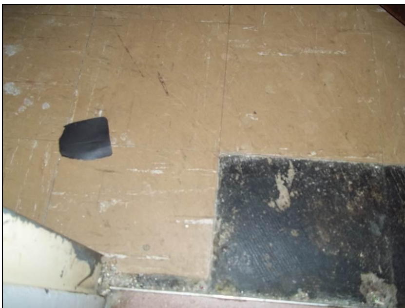
Photograph 4: Asbestos containing 9" x 9" vinyl floor tile, in fair condition (sample DH-16).
