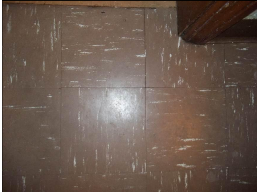
Photograph 5: Asbestos containing 9" x 9" vinyl floor tile, in fair condition (sample DH-18).
