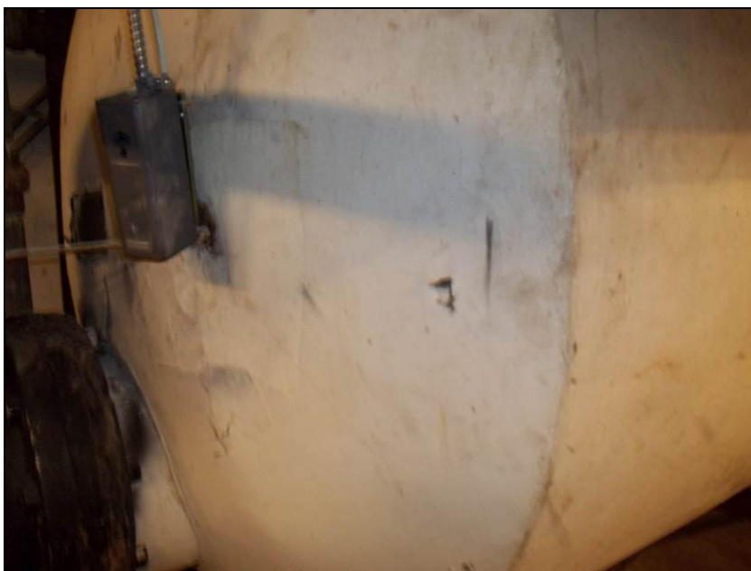
Photograph 2: Tank insulation in Room DH004A/004, in fair condition.
