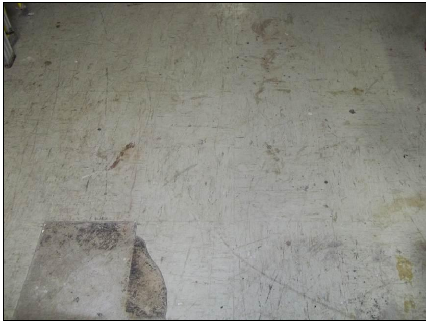
Photograph 13: Asbestos containing 1' x 1' vinyl floor tile.
