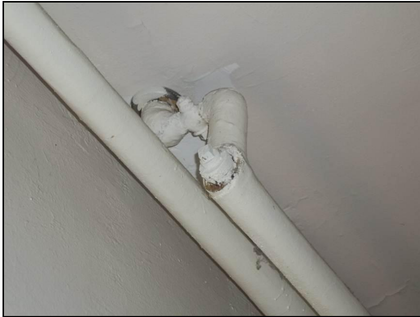
Photograph 5: Pipe fitting insulation in Stairway HA3S03, in poor condition.
