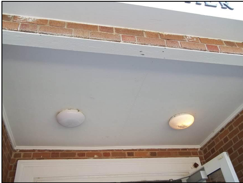
Photograph 19: Suspect asbestos containing transite ceiling panel (and asbestos containing light fixture heat shields, HA-6) exterior of the main entrance to the building.
