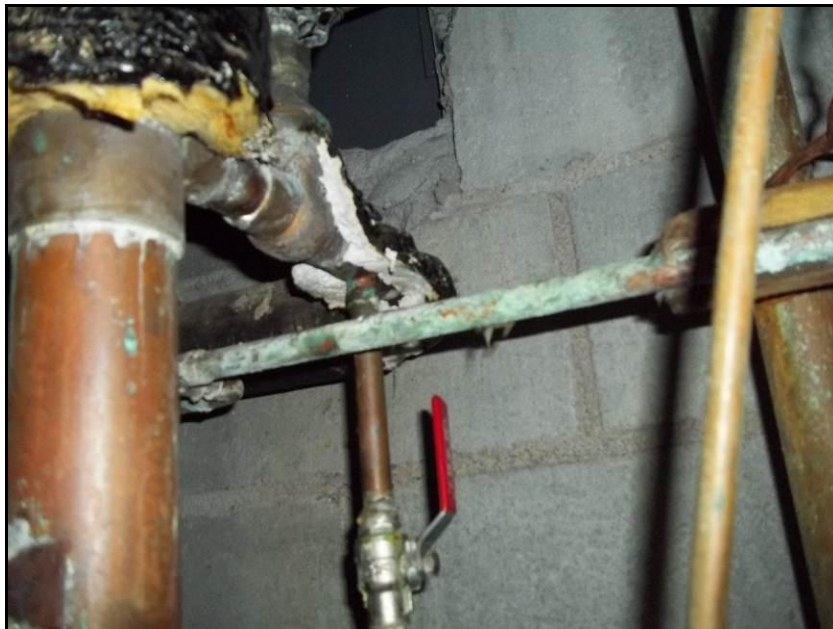
Photograph 6: Pipe fitting insulation in the access hatch in Room HA321, in poor condition.
