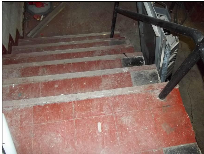
Photograph 18: Asbestos containing 9" x 9" vinyl floor tile, sample HA-35.
