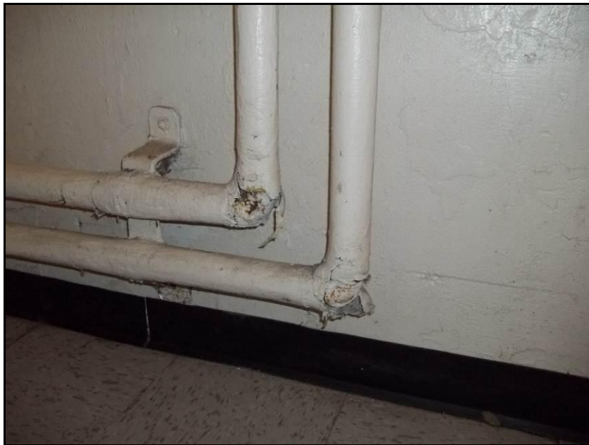
Photograph 2: Pipe fitting insulation in Stairway HA1S03, in poor condition.
