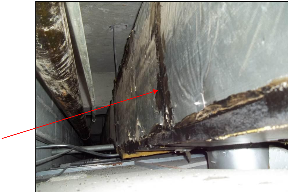
Photograph 11: Asbestos containing tar sealant on fiberglass duct above the ceiling tiles in Corridor HA1C02.
