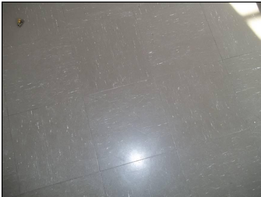
Photograph 14: Asbestos containing 9" x 9" vinyl floor tile, sample HA-1.
