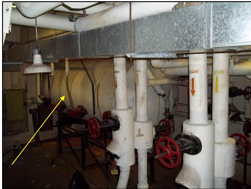
Photograph 10: Asbestos containing tank insulation in Room HA114.
