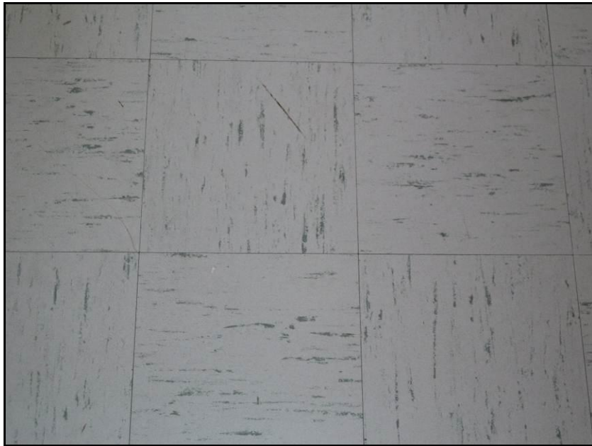
Photograph 15: Asbestos containing 9" x 9" vinyl floor tile, sample HA-4.
