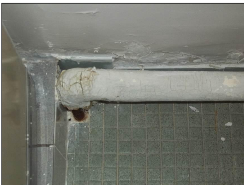
Photograph 8: Pipe fitting insulation in the shower of Room HA507 in poor condition..
