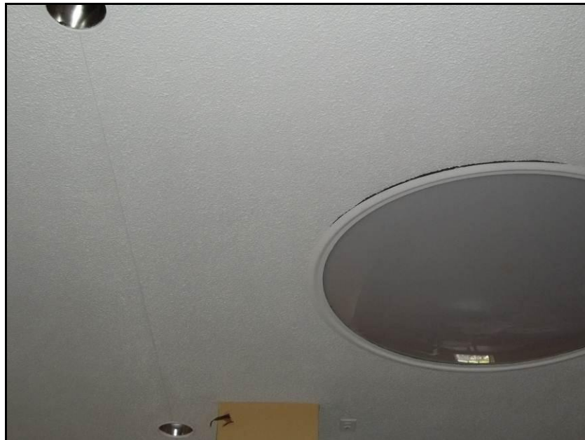
Photograph 12: Asbestos containing texture coat on the ceilings of HA210 and HA211.
