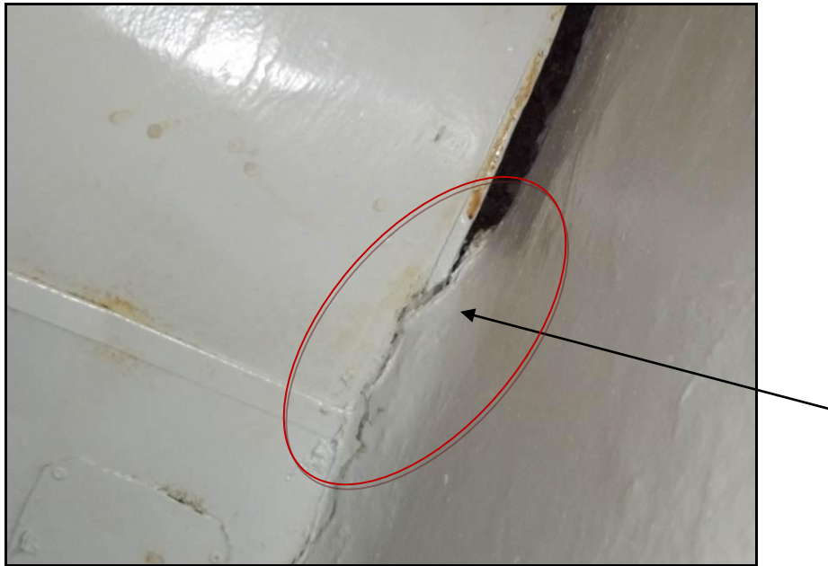
Photograph 9: Duct in Room HA208, too high to assess. As such it must be considered to be asbestos containing until proven otherwise.
