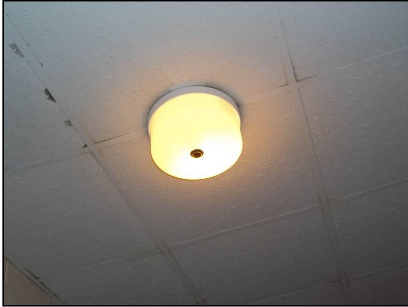
Photograph 21: Asbestos containing light fixture heat shields, HA-24.
