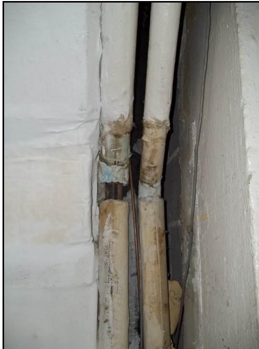
Photograph 4: Pipe fitting insulation in Room HA208, in poor condition.
