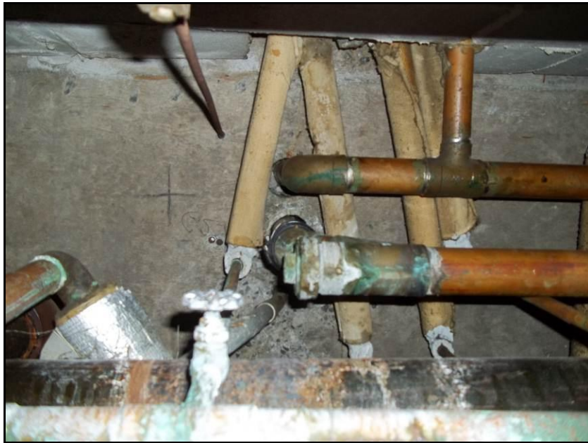
Photograph 1: Pipe fitting insulation in the Corridor HA1C03, in poor condition. Limited viewing was available above the ceiling tiles.
