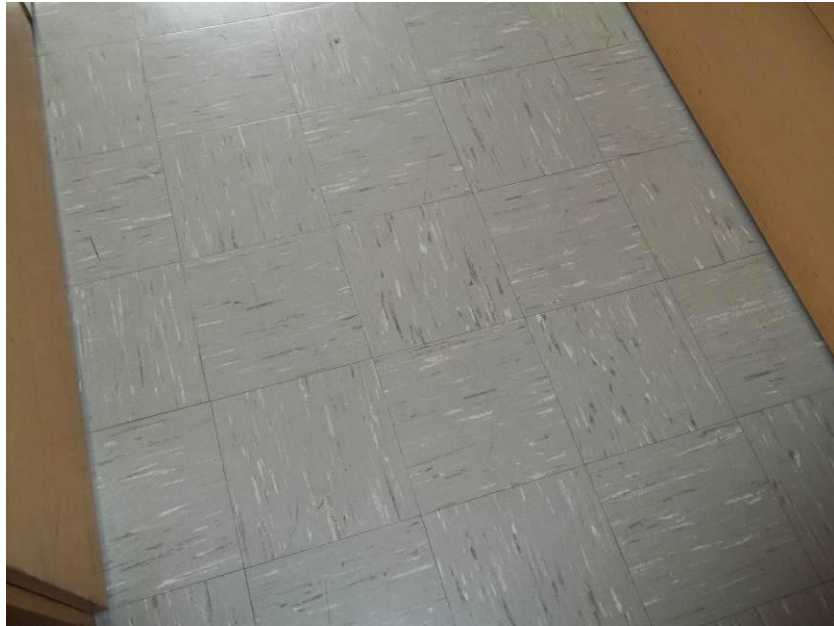
Photograph 17: Asbestos containing 9" x 9" vinyl floor tile, sample HA-15A
