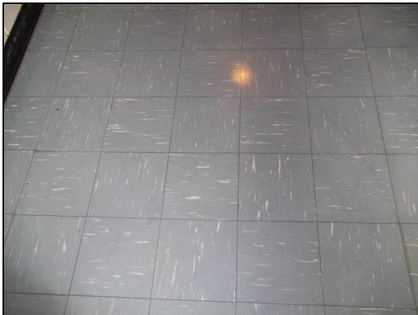
Photograph 16: Asbestos containing 9" x 9" vinyl floor tile, sample HA-13
