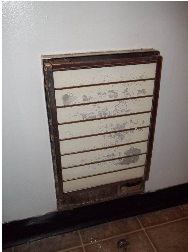
Photograph 11: Sample GB-11. The asbestos containing transite heater panel was found on select washroom walls.
