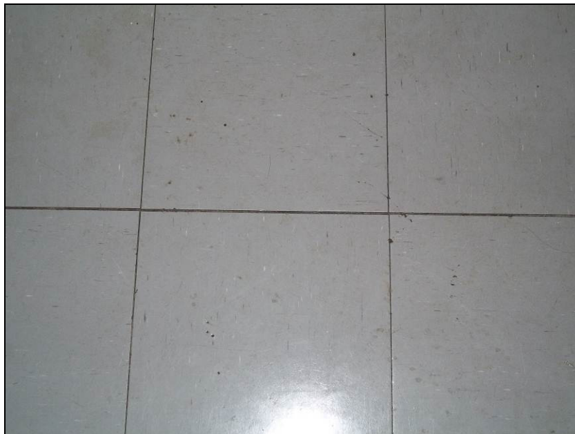
Photograph 10: Sample GB-25. The vinyl floor tile was identified as non-asbestos containing. The mastic was found to contain 2% Chrysotile asbestos.
