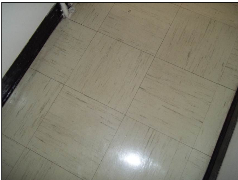
Photograph 6: Sample GB-6. Asbestos containing vinyl floor tile.
