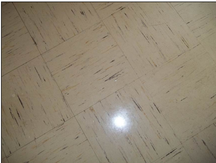
Photograph 5: Sample GB-1. Asbestos containing vinyl floor tile.
