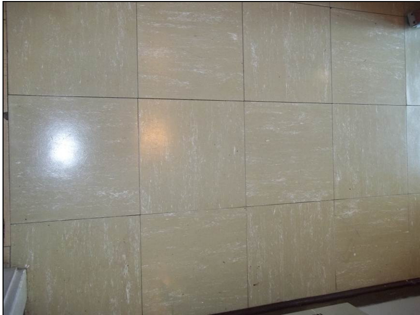
Photograph 9: Sample GB-24. Asbestos containing vinyl floor tile.
