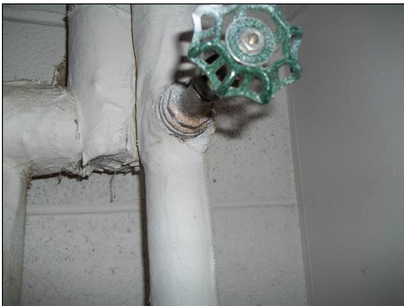
Photograph 1: Suspect asbestos containing pipe fitting insulation in Room GB202, in poor condition.
