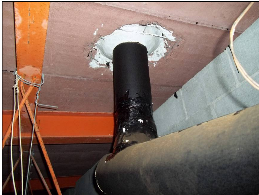
Photograph 10: One of three rain water leaders observed in the building. These were too high to access for sampling. As such, they must be considered to be asbestos containing until proven otherwise.
