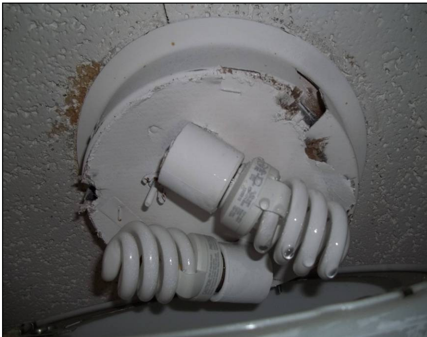
Photograph 8: Sample CU-7, damaged light fixture heat shield.
