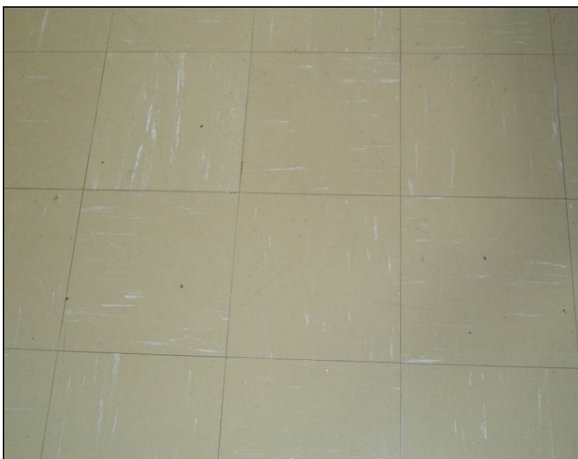
Photograph 5: Sample CU-13, yellow with white 9" x 9" vinyl floor tile.
