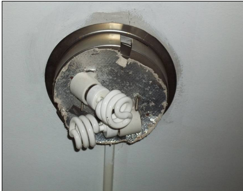
Photograph 9: Sample CU-10, damaged light fixture heat shield.
