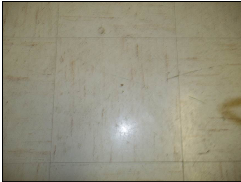
Photograph 3: Asbestos containing 1' x 1' vinyl floor tile (Sample CA-1).
