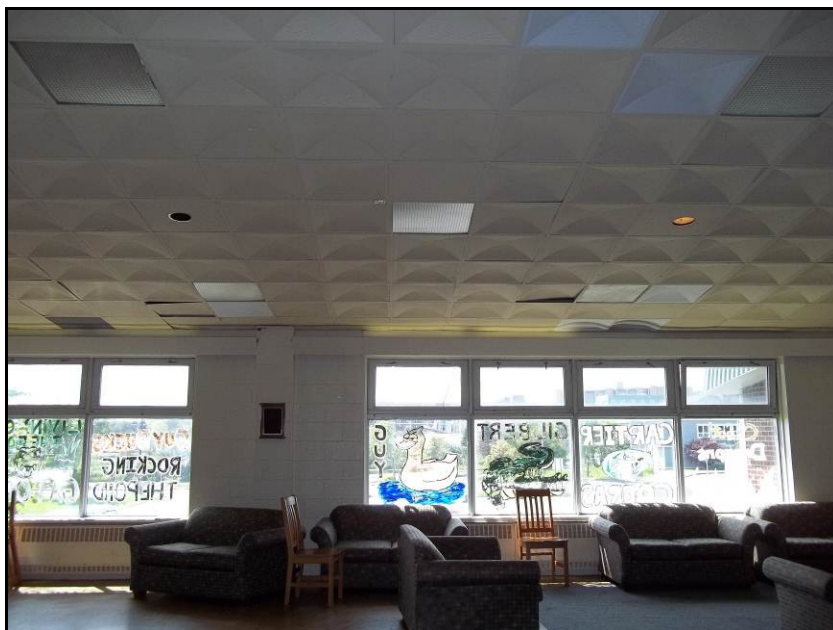
Photograph 1: Ceiling tiles of Room CA2000 were visually identified as a cardboard based tile.
