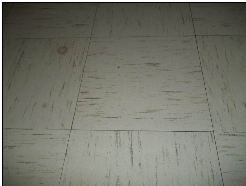
Photograph 5: Asbestos containing 1' x 1' vinyl floor tile (Sample CA-11).
