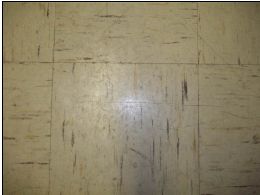
Photograph 4: Asbestos containing 1' x 1' vinyl floor tile (Sample CA-6).
