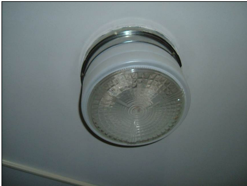
Photograph 18: Sample CR-29. Light globe associated with asbestos containing light fixture heat shield.
