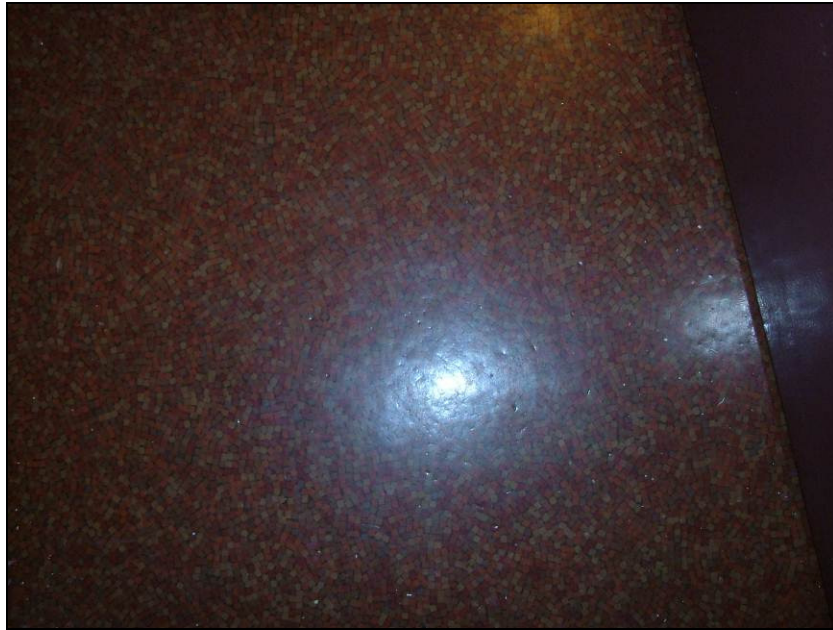
Photograph 5: Sample CR-9, asbestos containing vinyl sheet flooring.
