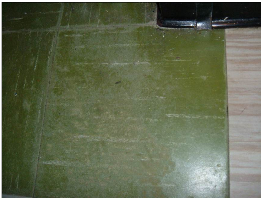
Photograph 8: Sample CR-5 asbestos containing vinyl floor tile and mastic.
