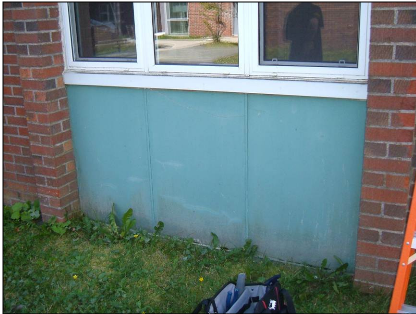
Photograph 15: Sample CR-34. Asbestos containing transite panels at the exterior of the building. Suspected to be similar material on all exteriors of Burtons Pond residences.
