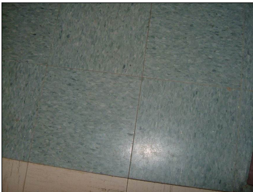
Photograph 12: Sample CR-22 asbestos containing mastic associated with the non-asbestos containing tile.
