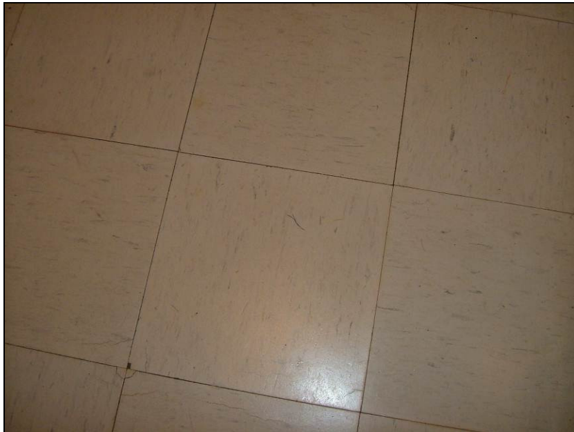
Photograph 14: Sample CR-33 asbestos containing mastic associated with the non-asbestos containing tile.
