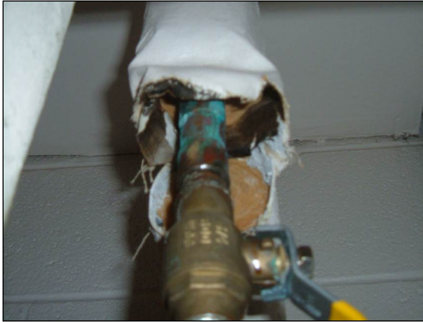
Photograph 1: Pipe fitting insulation debris in the closet of Room CR209, in poor condition.
