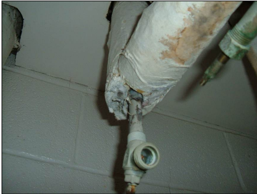
Photograph 3: Pipe fitting insulation debris in the closet of Room CR108, in poor condition.
