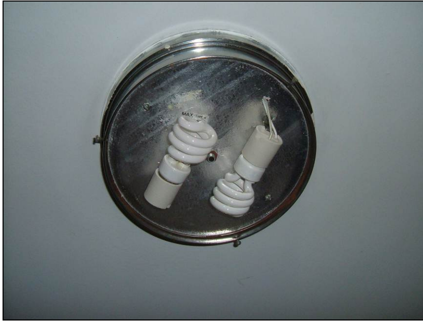
Photograph 17: Sample CR-29. Asbestos containing light fixture heat shield.
