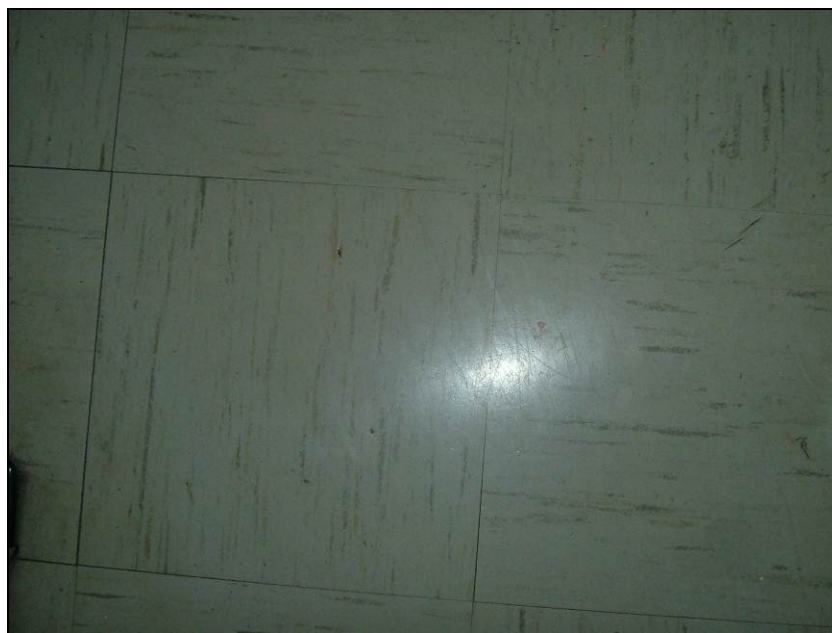
Photograph 10: Sample CR-8 asbestos containing vinyl floor tile.
