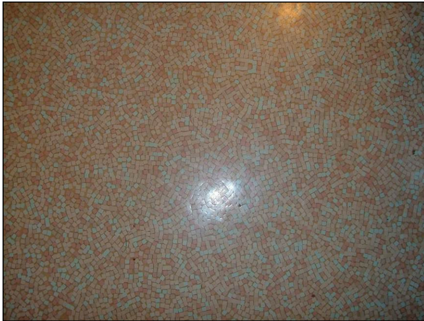
Photograph 4: Sample CR-4, asbestos containing vinyl sheet flooring.
