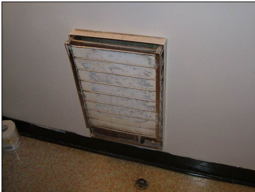
Photograph 16: Sample CR-16. Asbestos containing transite on heaters in washrooms.
