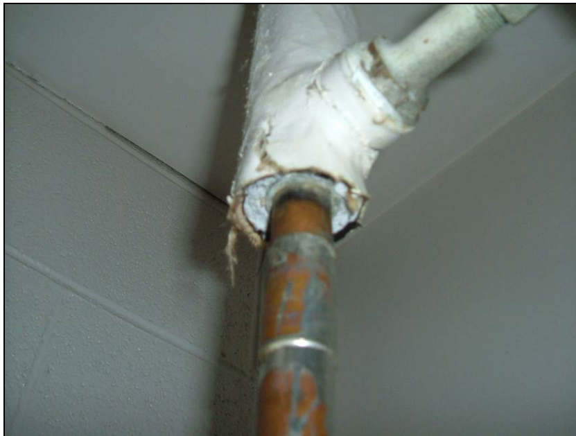
Photograph 2: Pipe fitting insulation debris in the closet of Room CR210, in poor condition.
