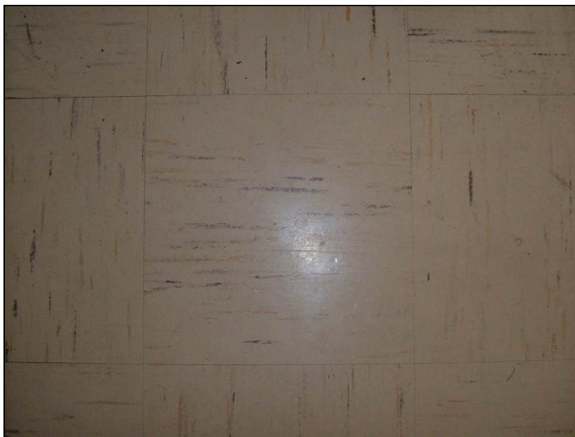
Photograph 7: Sample CR-1 asbestos containing vinyl floor tile and mastic.
