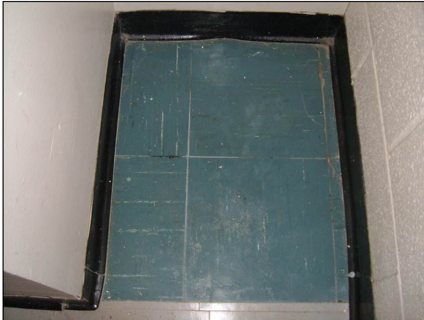
Photograph 13: Sample CR-28 asbestos containing vinyl floor tile and mastic.
