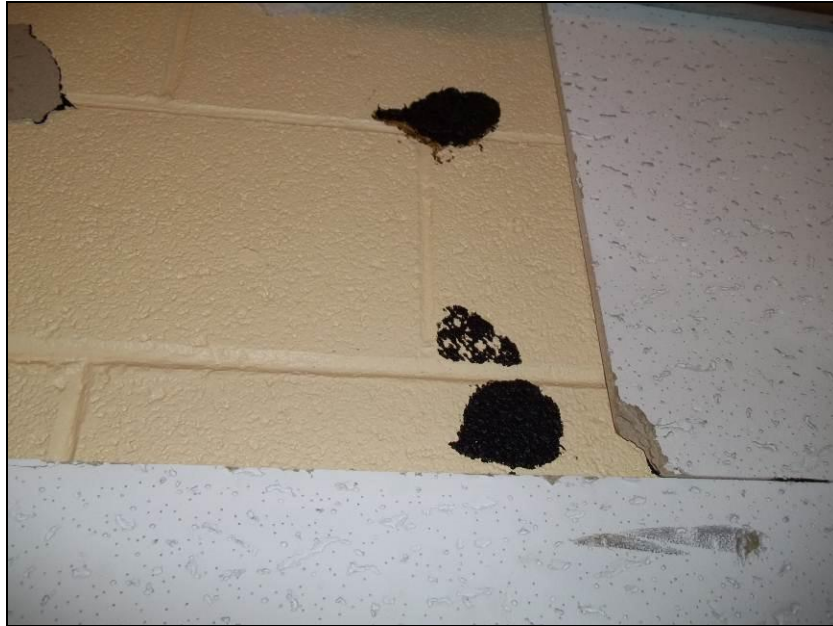
Photograph 3: Sample CT-16. Asbestos containing ceiling tile adhesive on the walls of Room CT312.
