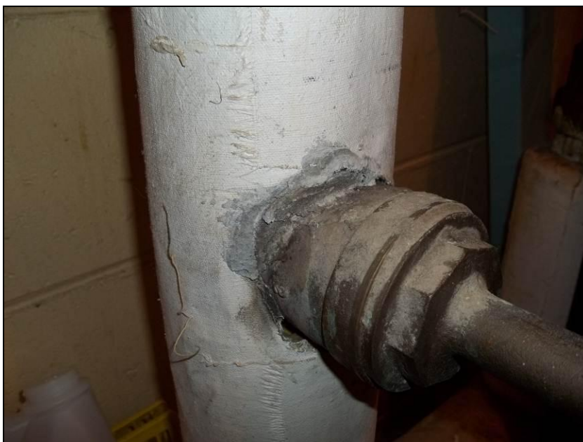
Photograph 2: Suspect asbestos containing pipe fitting insulation in Room CT112, mechanical room, in poor condition.
