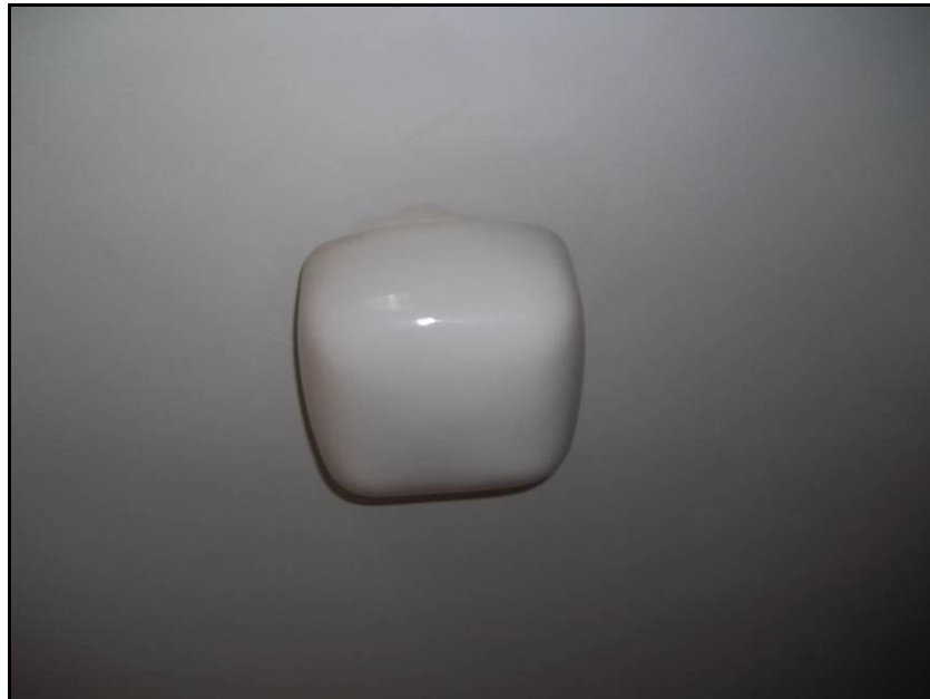
Photograph 18: Sample CT-12. Globe associated with asbestos containing light fixture heat shield.
