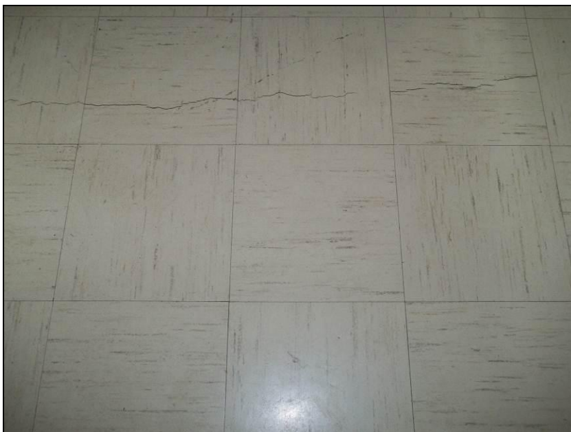
Photograph 12: Sample CT-13. The vinyl floor tile was found to contain 8% Chrysotile asbestos.
