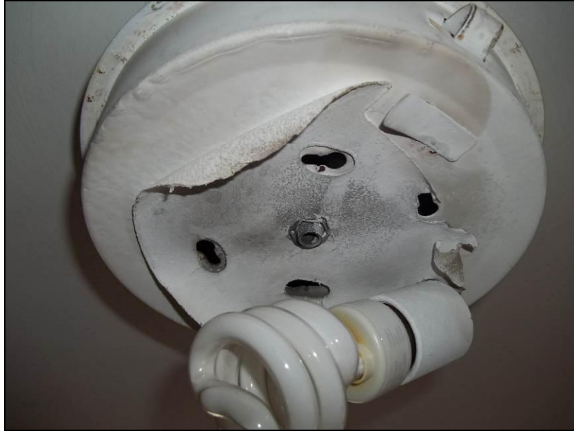
Photograph 17: Sample CT-12. Asbestos containing light fixture heat shield.
