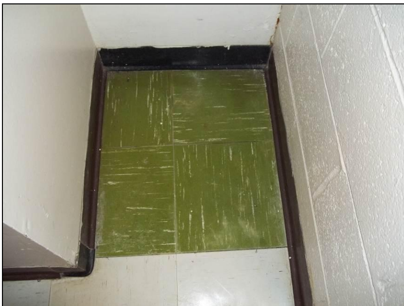
Photograph 14: Sample CT-23. The vinyl floor tile was found to contain 8% Chrysotile asbestos, and the mastic was found to contain 3% Chrysotile asbestos.
