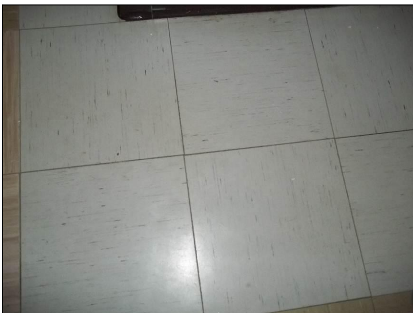
Photograph 13: Sample CT-20. The vinyl floor tile was identified as non-asbestos containing. The mastic was found to contain 3% Chrysotile asbestos.
