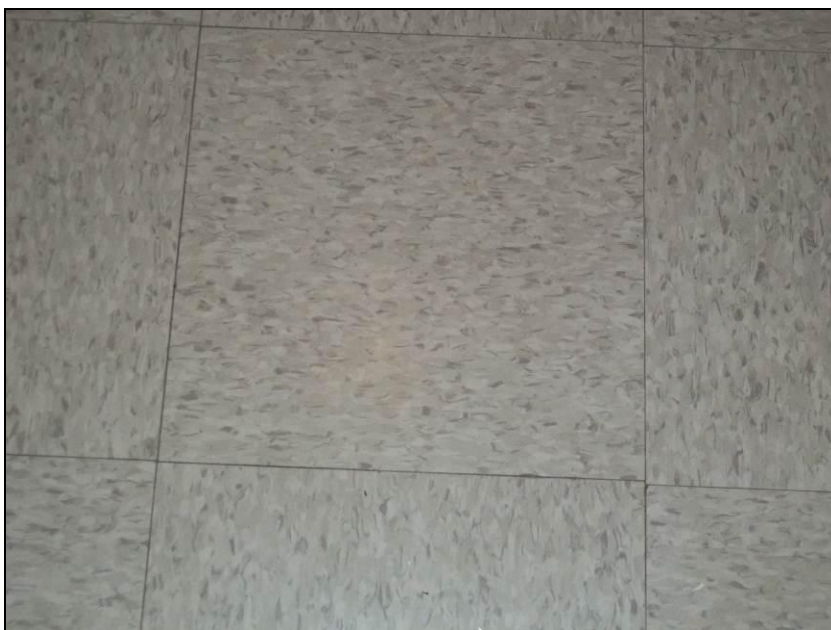
Photograph 8: Sample CT-2. The vinyl floor tile was identified as non-asbestos containing. The mastic was found to contain 5% Chrysotile asbestos.
