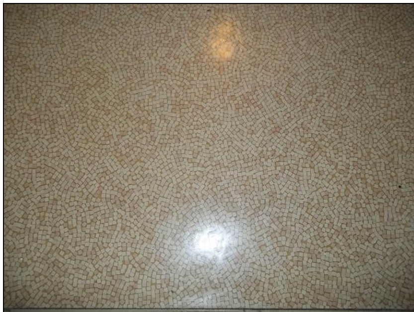
Photograph 5: Sample CT-8. The flooring was found to contain 20% Chrysotile asbestos.
