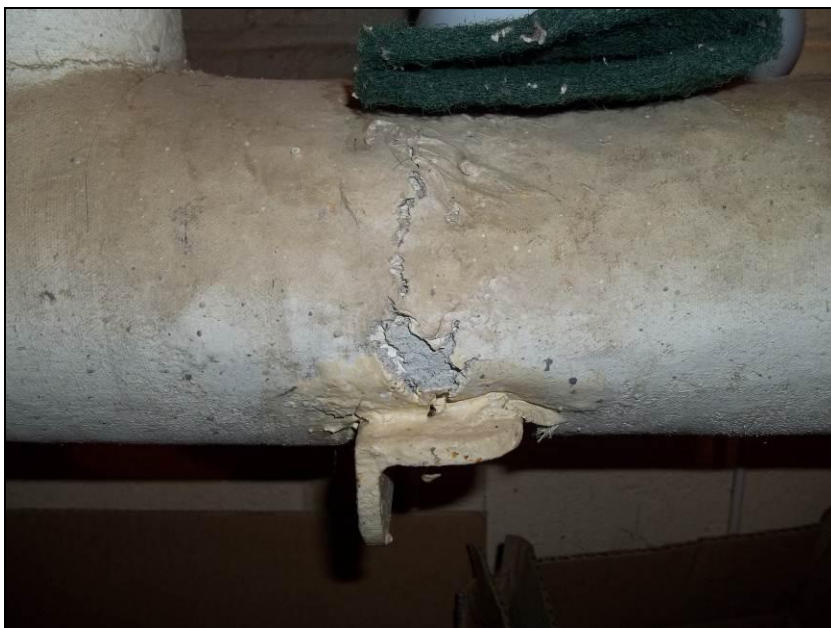
Photograph 1: Suspect asbestos containing pipe fitting insulation in Room CT112, mechanical room, in poor condition.
