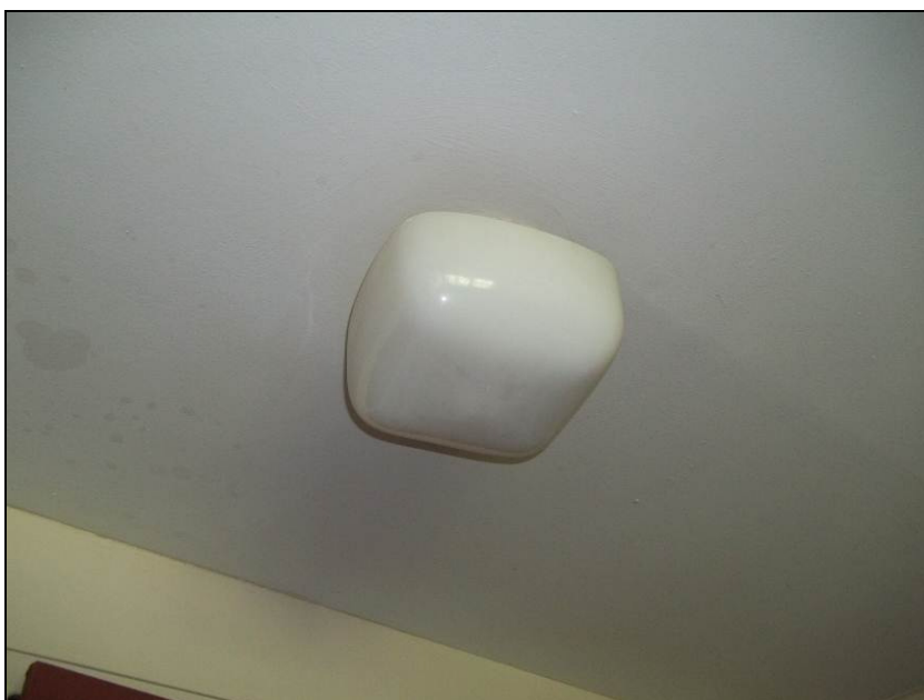
Photograph 5: Light fixture heat shield, containing 15% Chrysotile asbestos. Sample BM-9
