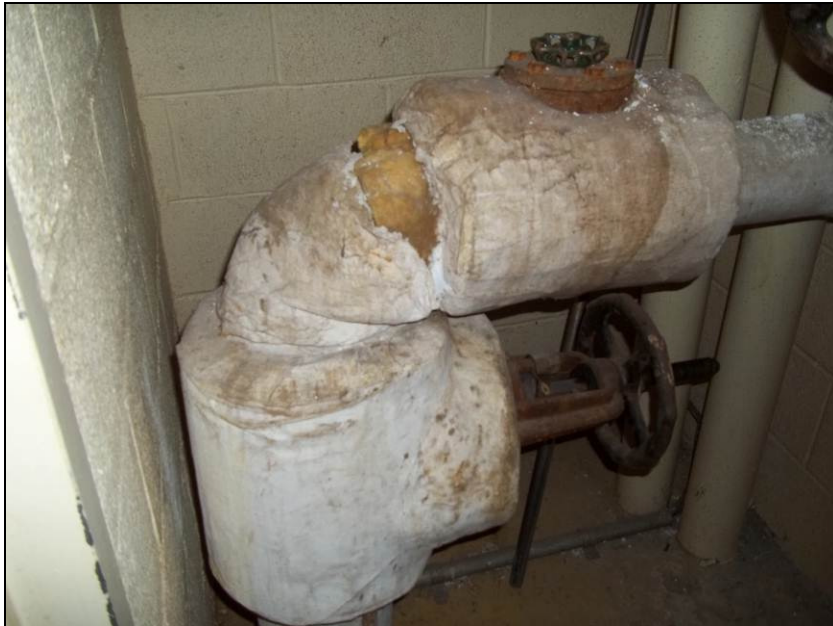
Photographs 1: Room BM106. Pipe fitting insulation in poor condition
