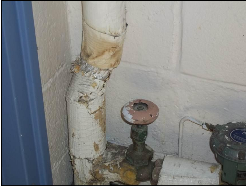
Photograph 1: Pipe fitting insulation in the Corridor DO3C01, in poor condition.
