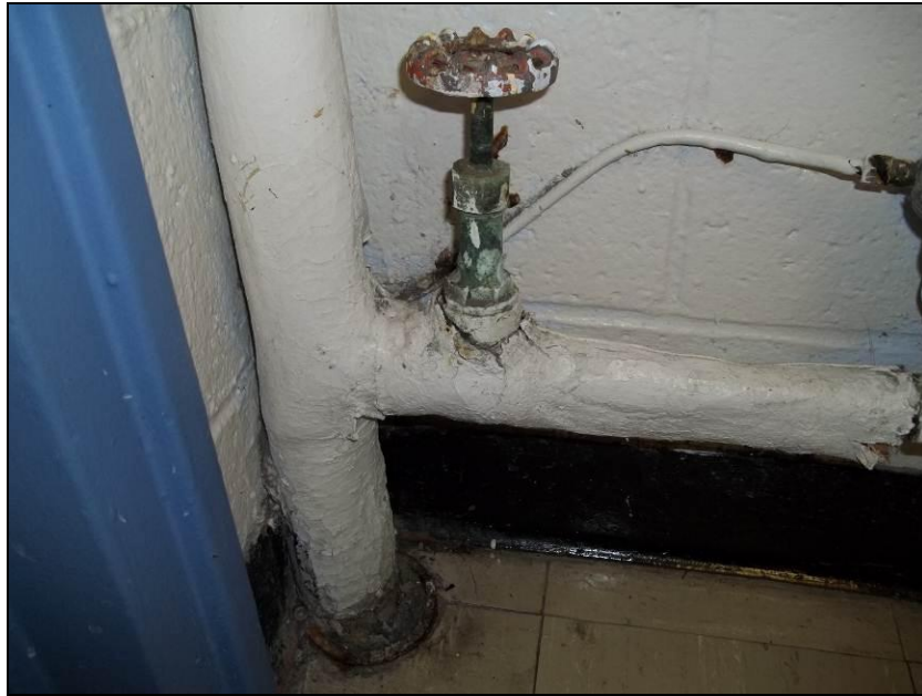
Photograph 3: Pipe fitting insulation in Room DO216, in poor condition.
