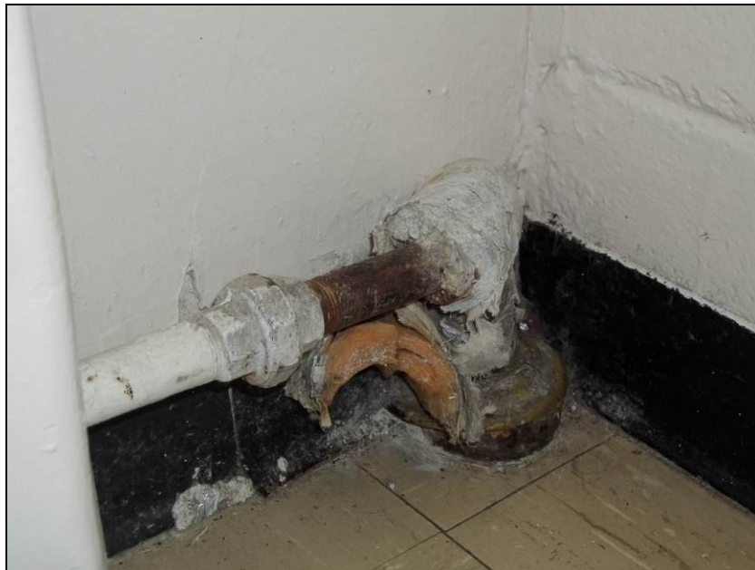
Photograph 4: Pipe fitting insulation in Corridor DO4C01, in poor condition.
