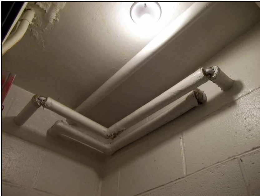
Photograph 2: Pipe fitting insulation in Room DO216, in poor condition.
