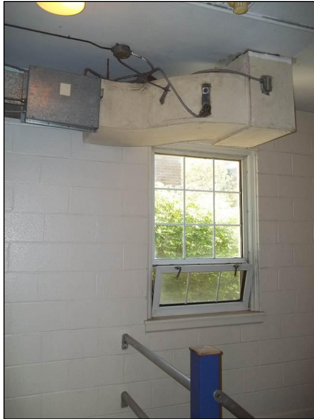
Photograph 9: Insulation duct located above a stairway of DO1S03. The duct was not accessible for sampling. As such it must be considered to be asbestos containing until proven otherwise.
