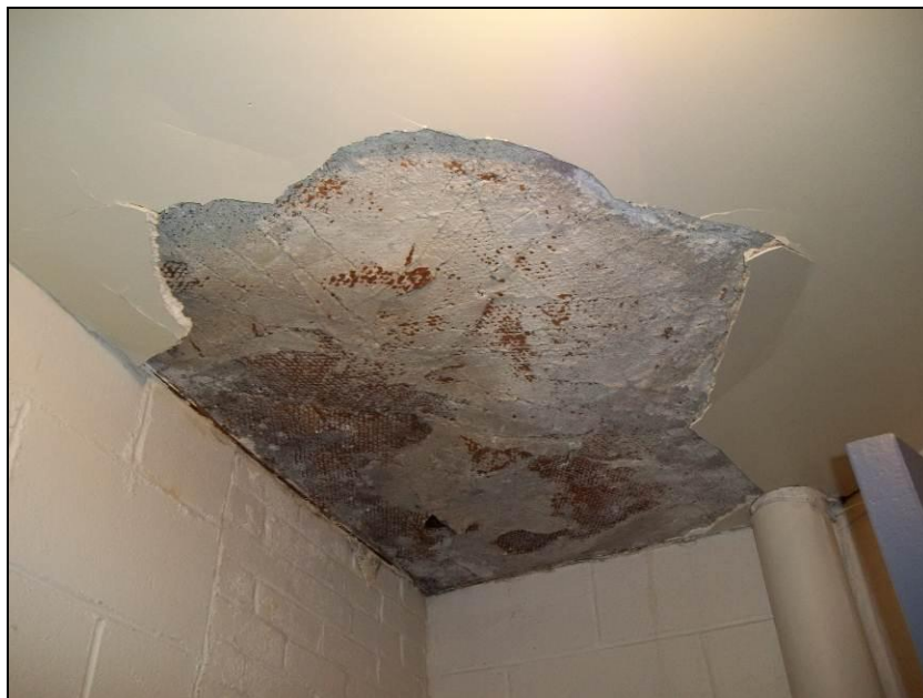
Photograph 8: Sample DO-21, as found in Room DO409. The plaster is in poor condition.
