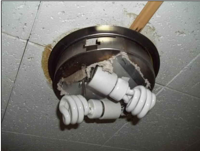
Photograph 7: Sample DO-13 as found in Room DO111. Light fixture heat shield in poor condition.
