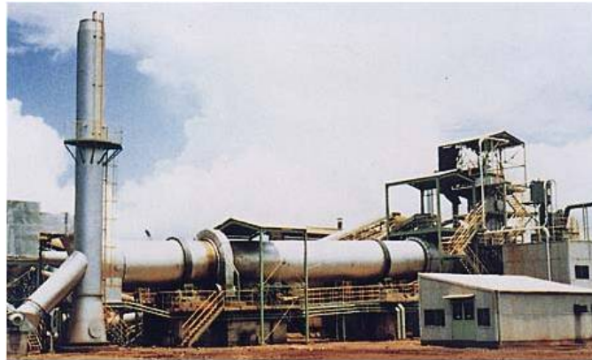
Figure 5: Photograph of a rotary dryer.
