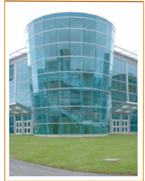
Inco Innovation Centre
